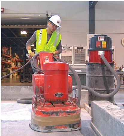
Worker milling granite floor indoors with milling machine and dust collection system Photo credit: OSHA
