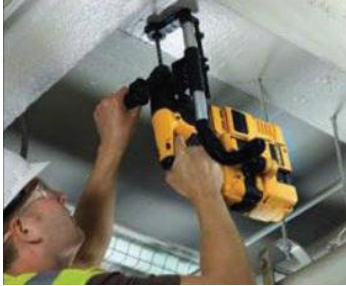
Worker drilling into concrete with a rotary hammer equipped with shroud and dust collection system. Note the shroud around drill bit, silver and black hose, and dust collector are attached conveniently to the drill Photo credit: DeWalt & OSHA
