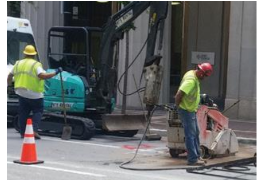
Walk-behind saw with water delivery system Photo credit: OSHA
