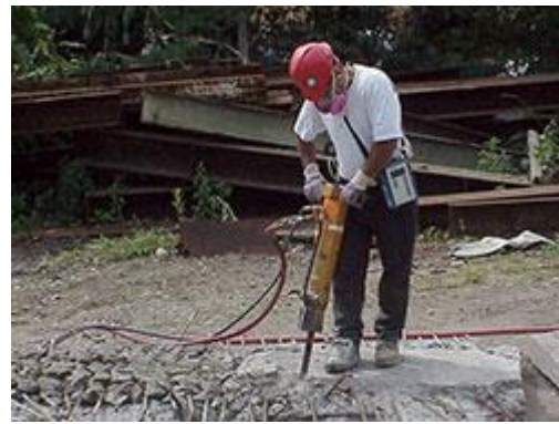
Jackhammering with water-spray control to reduce dust Photo credit: NIOSH
