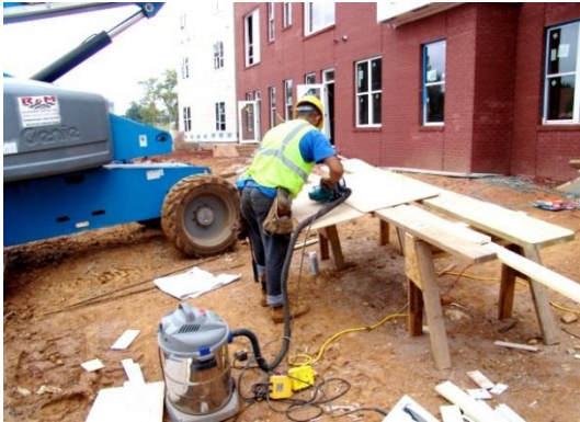
Cutting fiber cement board using circular saw with HEPA Vac Photo credit: NIOSH
