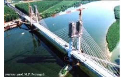
High speed railway bridge over the Po river
