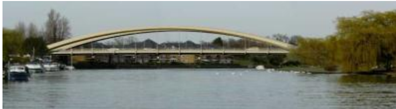
Walton Bridge – Surrey County Council
