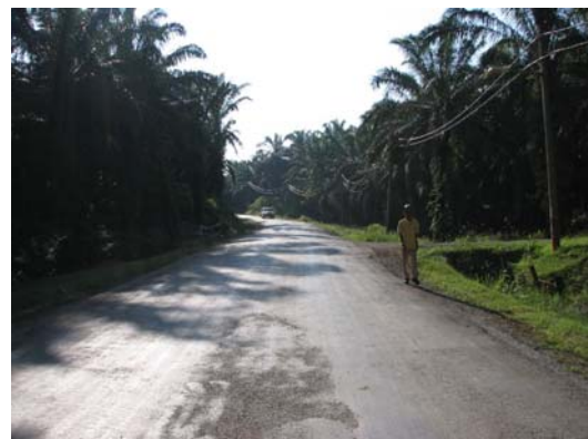
Plate 5: Upgraded Access Road at Tun Tan Estate
