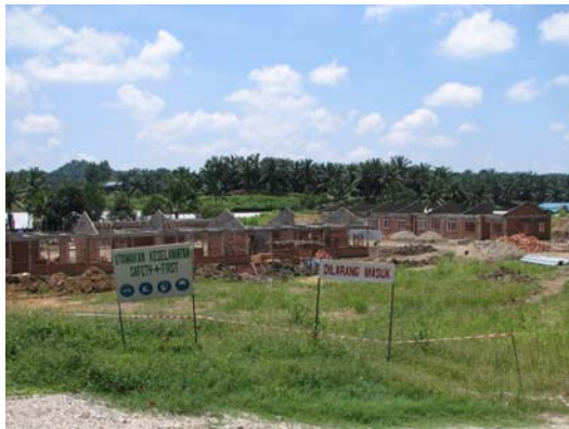
Plate 2: Housing Under Construction
