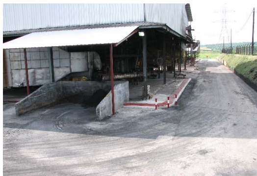
Plate 2: Very Good Facility for Storage of Boiler Ash at Sedenak Mill, January 2010
