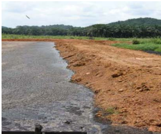
Plate 3: Recent Earthworks to Increase the Effluent Pond Freeboard
