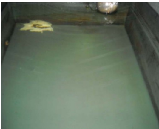
Plate 2: Overhead Household Water Tank after Cleaning
